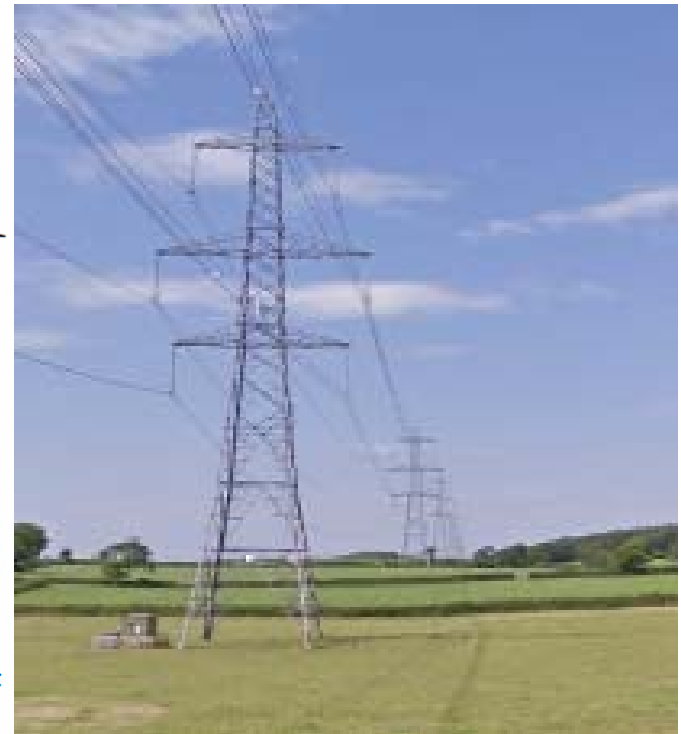
400kV double circuit
